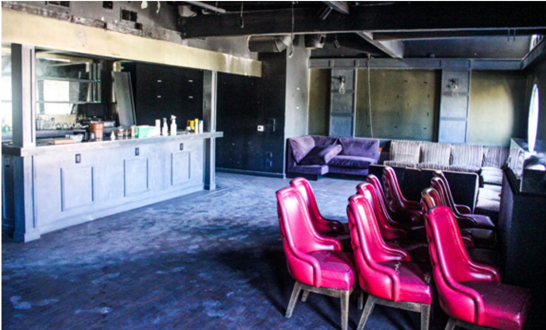
Second Floor Bar / Office
